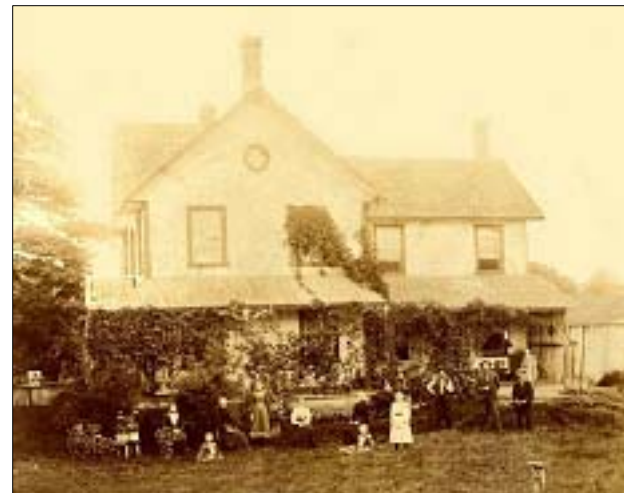
Older view of the east side of the house
